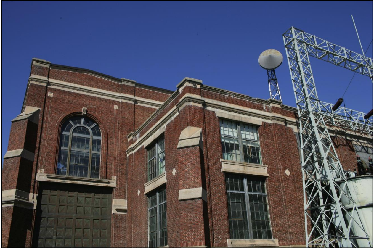
Figure 2.3-5. Bellows Falls powerhouse.
